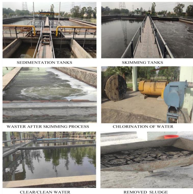
**FIGURE 3.4:** Primary and Secondary treatment
